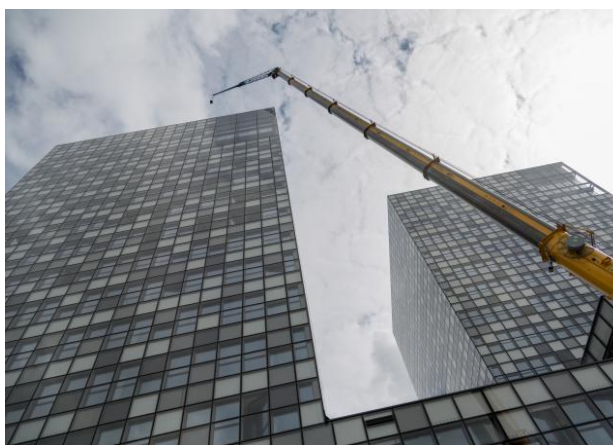
Fig. 3: Construction of a new office building in Luxembourg City
